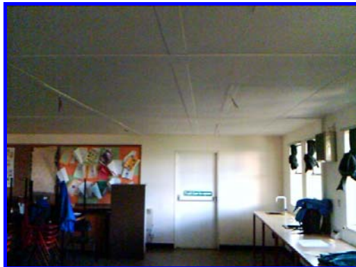
X4 showing finish walls & ceilings
