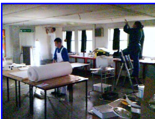
X4 Classroom insulation work
