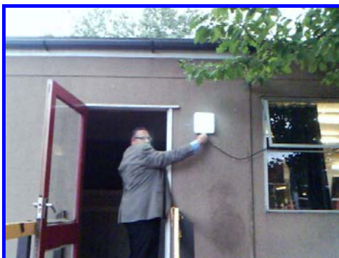
External trials of the LED replacement.
