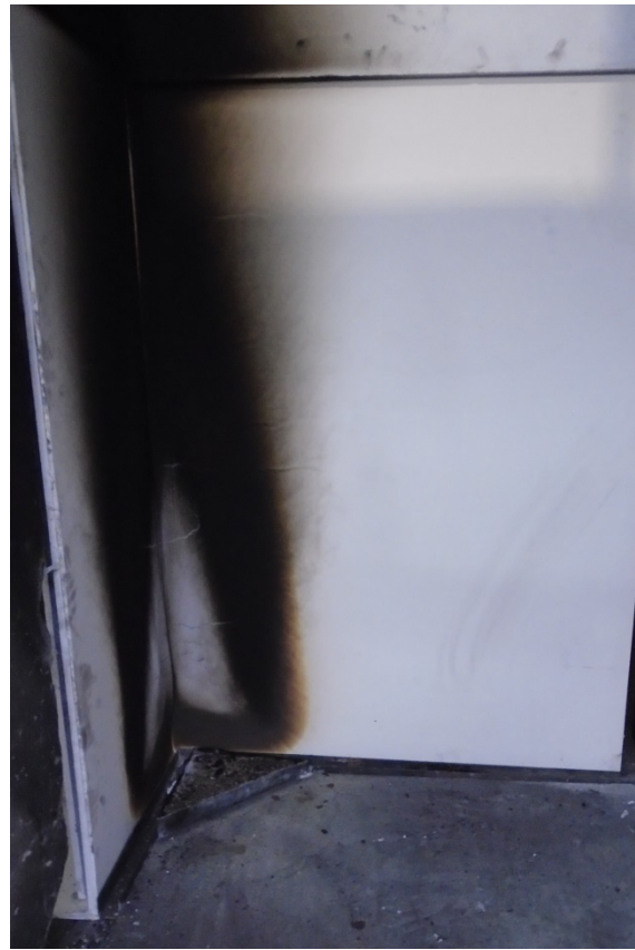
Figure 8: Total view of the exposed surface of the long wing after testing
